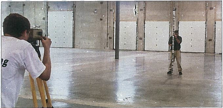
Using a digital level and bar-coded rod, Chris Harding and Mike Fischer get very accurate readings. The measurements verify the 3-D scans. PHOTO: NASVIK
