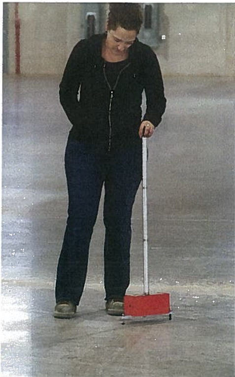
Becky Kazmierski with H.H. Holmes Testing Laboratories uses a D-Meter to measure curling in floor panels.
