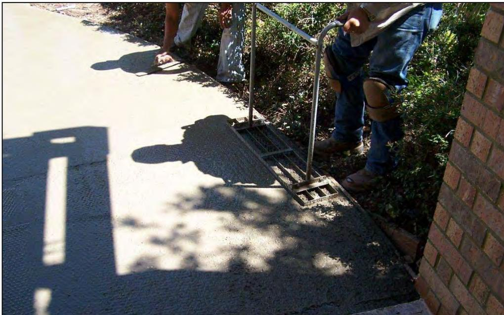
**Jitterbugging helps minimize fiber appearance on stamped concrete.**
