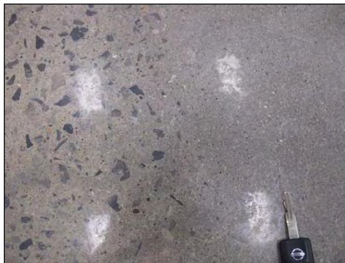
**Fiber evidence disappears once grind depth goes through the surface paste**
