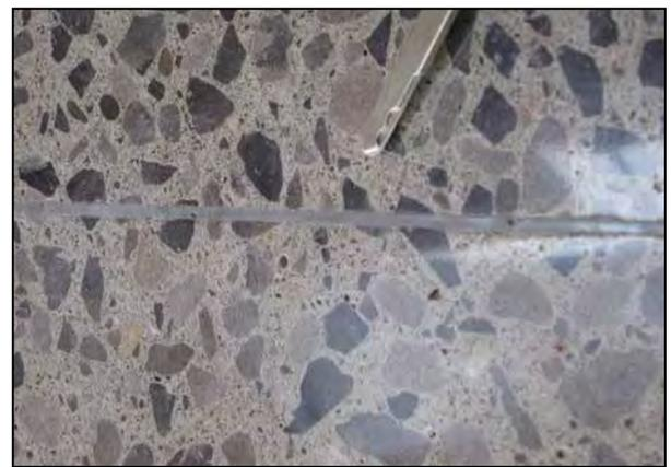
**Deep aggregate grind eliminates fiber appearance**
