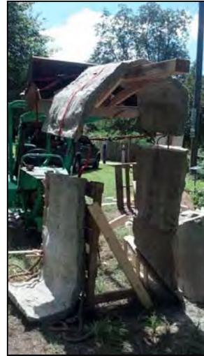
**Concrete formed in panel segments and assembled**
