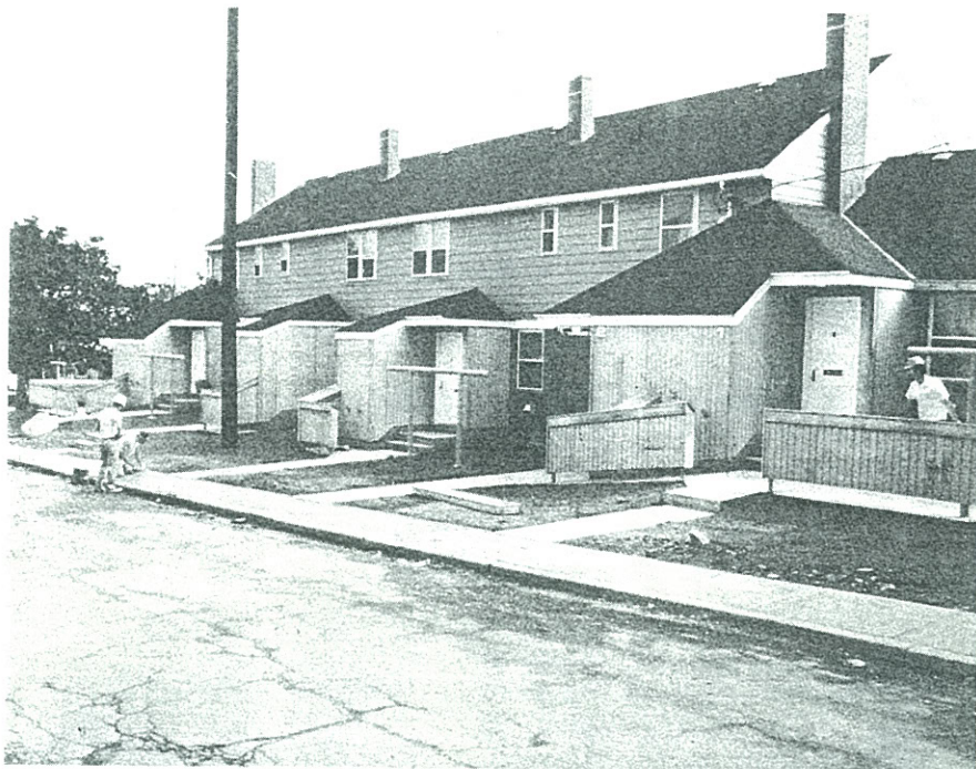
Fig. 2 — Harbor Homes housing project, Erie, Pa., used polypropylene fibers in the curbs, sidewalks, and steps.
