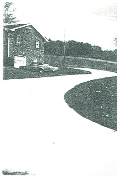
Fig. 3 — Fibrous reinforcement conforms to forms.
