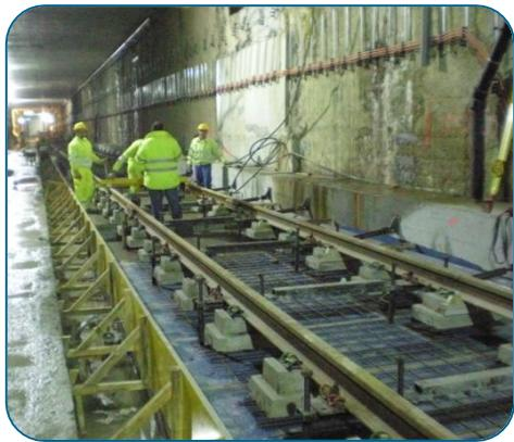
Example of a complete lay for a floating slab track
