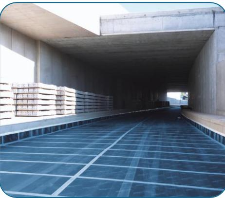
Example of a complete lay for a ballast track
