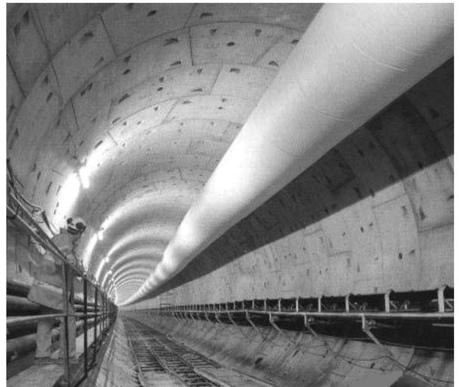
Fig. 5.1—Channel Tunnel Rail Link tunnel lining made with SFRC.
