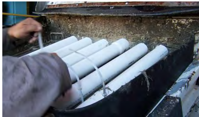
PVC pipe lay-over being zip-tied into place between slats.
