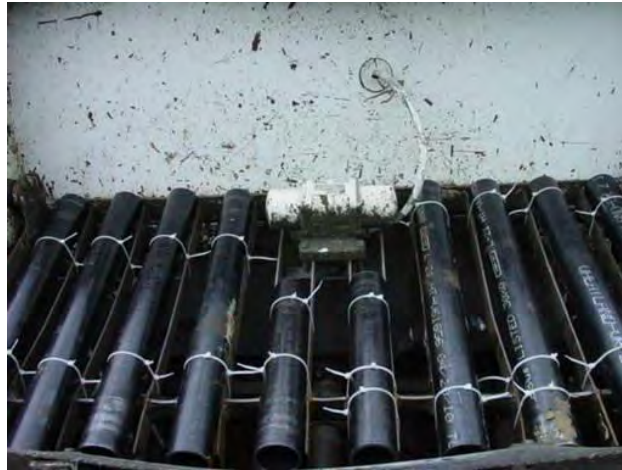
Metal pipe lay-over method zip-tied in place.
