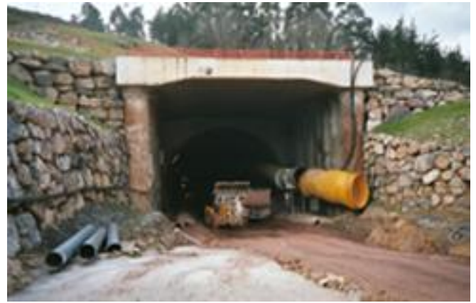
Over 30,000 lbs. of FORTA-FERRO ® fiber were used to line a tunnel for the city of Navarre, Spain.
