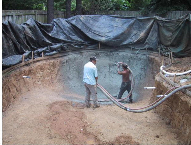
FORTA-FERRO® reinforced swimming pool – Germantown, TN
