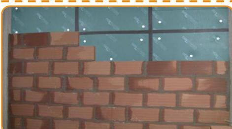
Build up the second wall by caring to joint the blocks with mortar on both vertical and horizontal joints.
