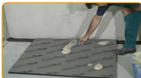
Apply the glue on the panel by spreading it on dots.
