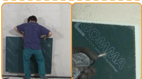
Place the panel on the right wall position and produce 5 holes per panel with the driller (one in the centre and one in the four corners)
